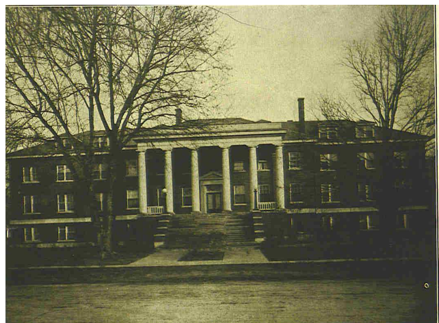
Denhart Hall - Completed in 1918, the building was the largest girls' dormitory on the campus. The building was destroyed by fire in the spring of 1980.
