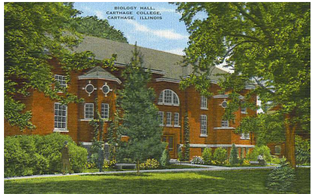
The first gymnasium, later Biology Hall, was home of the revered Biology Department at Carthage College. This building is scheduled for demolition.
